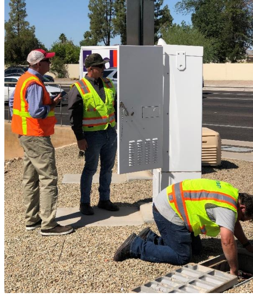
Scottsdale traffic technicians checked each cabinet and conduit pull box at the intersections along Hayden Road.
